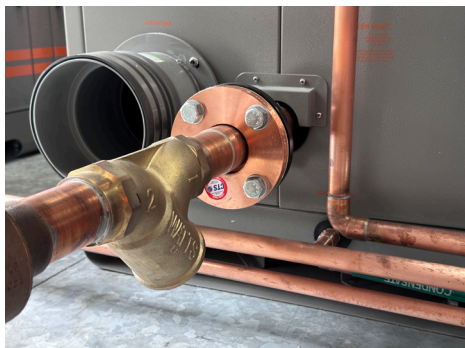
Copper Coated out of equipment to Y strainer
