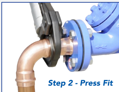
Use the simple, quick Press Fit method
