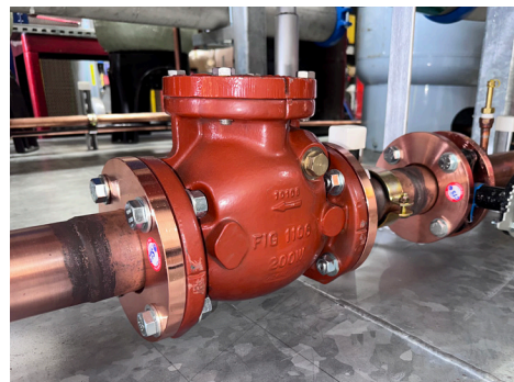
Copper Coated flange to check valve
