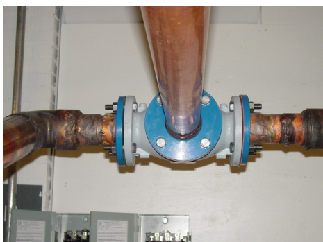
High pressure heavy gauge 150lb divertor valve
