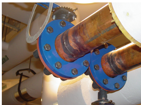
High Pressure mains water supply to main generator
